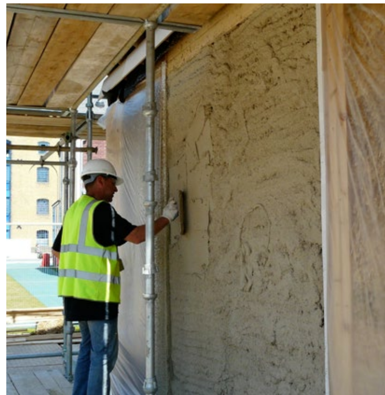
Fig 2 Lime Rendering of a ModCell® Panel
