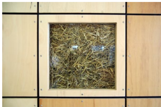
Fig 1 A truth window in a ModCell® Panel
